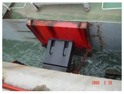
Aviation Fuel Supply Company Sha Chau Plant 香港航煤供应营运有限公司 Under the AFSC regular "Fender Renewal Plan", an 8 years old Trellex fender, condition of paint was still O.K.
